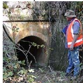
One of the concrete culverts - all in excellent condition
