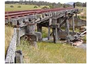
The transom top timber girder br. spanning Snakes Valley Creek
