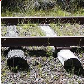
Some of the original "roundback" sleepers (possibly 1923)
