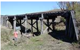
The transom top timber girder br. spanning Emu Valley Creek
