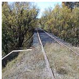
Fish River bridge
