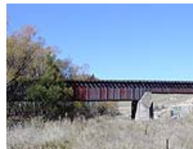
Southern half of the Fish River Bridge
