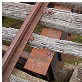
Plate web girder from the top showing the weathered transoms
