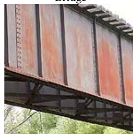
Plate web girder bracing.
