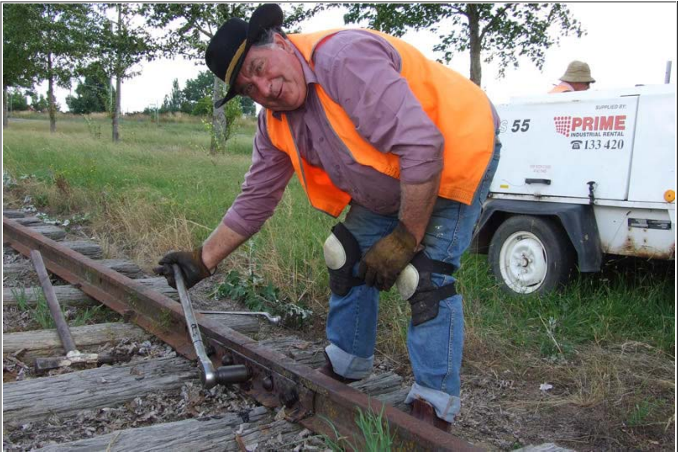
Replacing and greasing the fishplates is a messy job. Clive Payne does the preliminary tightening with a socket.
