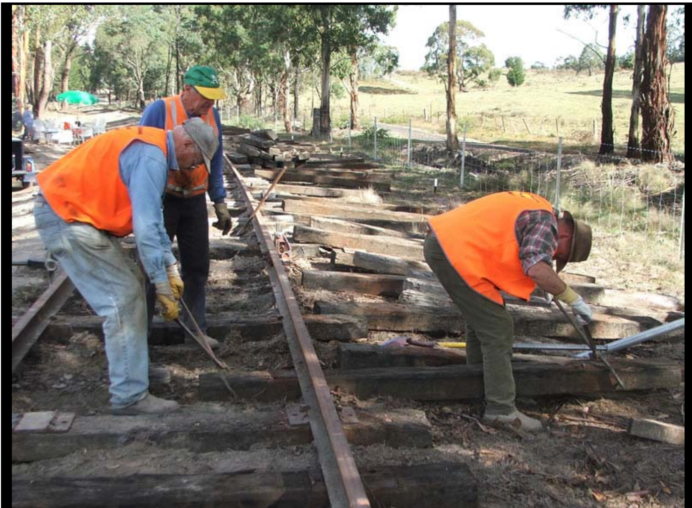
Head down & bum up was the procedure when dragging sleepers into place - we joked about being part of "Team Geriatric"
