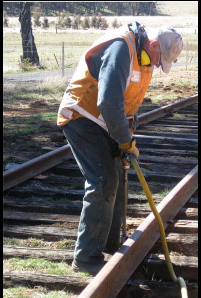
...and here on a pneumatic drill.
