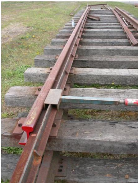
flanges are aligned within the groove. The check rails have been constructed by Moorhead Engineering to a standard State Rail design.
