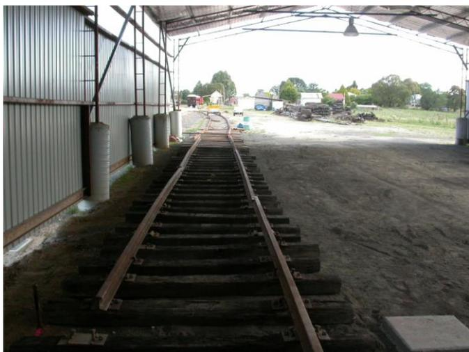
The photo above shows the view looking south towards the station from the interior of the shed, with the rail and sleepers in the process of being laid.
