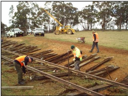
OTHR workers remove sleepers in the days **before** Oberon Council loaned OTHR the excavator (now with a sleeper grab) which has helped to speed up & lighten the work.
