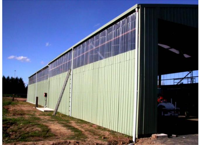
The March Working Bee saw some progress on the final tasks needed to complete the Rolling Stock shed. As can be seen in the photo above, the guttering and downpiping is all but complete. The Council has connected the water to the recently installed fire hoses, so these are now operational. We expect that the inspection by Oberon Council will take place shortly and our "Certificate of Occupancy" will be granted.
