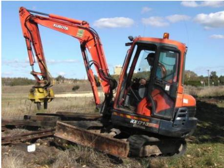
*Our Track Manager, Peter Culley removing and replacing sleepers with the sleeper grab.*
