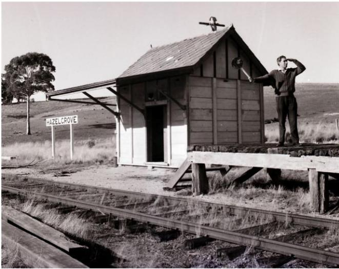
method of signalling the train to stop at Hazelgrove – hold out the green disc which was chained to a post at the station. The details of the rough and ready timber “platform” can be readily seen.
