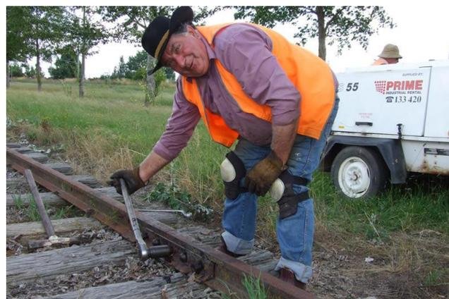
*Clive does the preliminary tightening of a fishplate with a socket*
