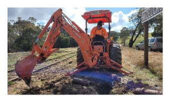
Hazelgrove - The original ceramic pipes were blocked and had to be removed in order to get storm water away from the track
