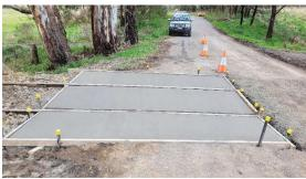
The Tip Road is another level crossing taking shape. This road needed to be kept open, so the crossing was poured in two parts.
