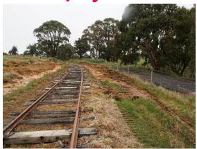
A view of the line showing drainage works to the left of picture. At this point there was quite a lot of flooding of the line.
