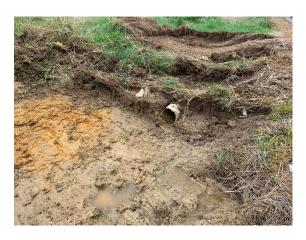
Work on the cess uncovered buried pipes which when cleared made a big difference
