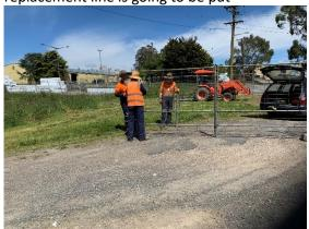
Survey and pegging out of the exact location of where the track will be located. This was done by Ontrack Survey & Design Pty Ltd
