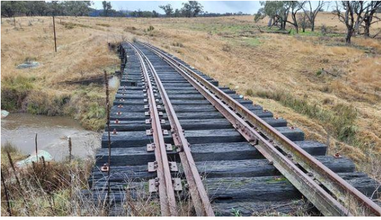
Looking across the Snakes Valley Creek bridge. Photo Michael Clark
