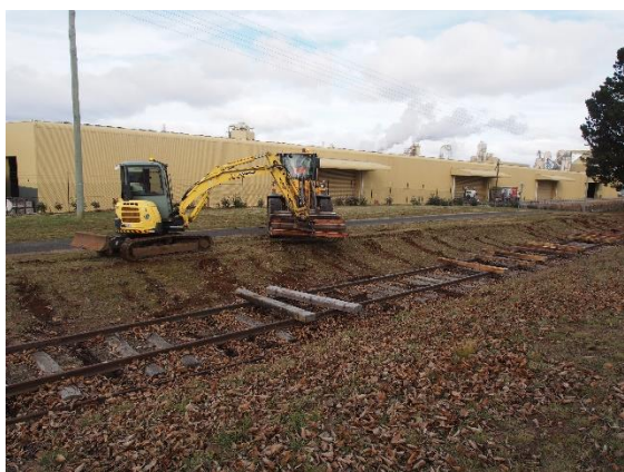
Sleeper removal and replacement near gate 6 of the Borg Factory
