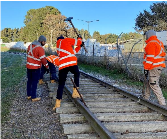
CAM workers doing some preliminary work to the track
