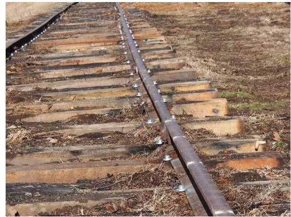
New sleepers in and screwed at Hazelgrove
