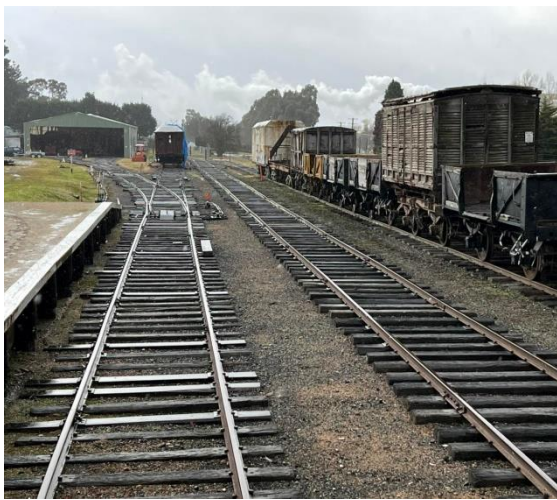
Looking down the line
