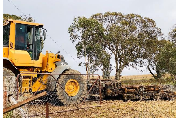
Old sleepers removed from the track and stacked.”
