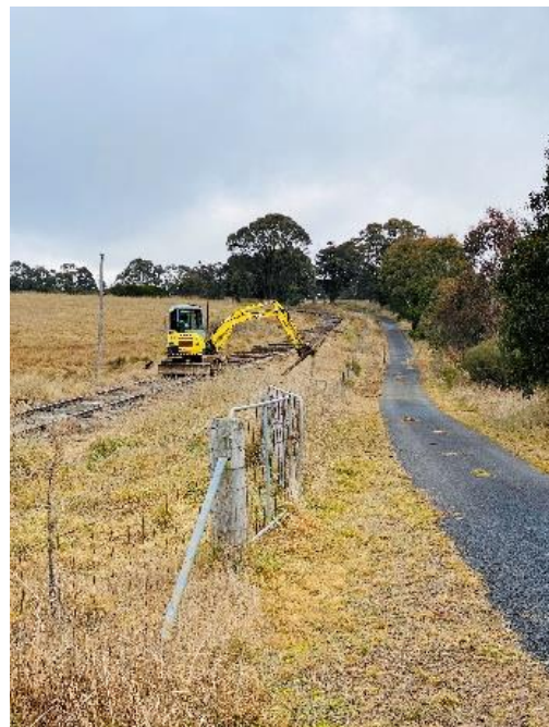
Track work underway with the walking track beside.
