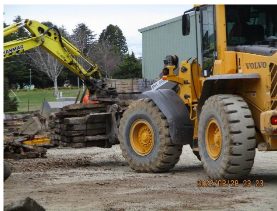
Contractors working in the security yard, Oberon Station Precinct.
