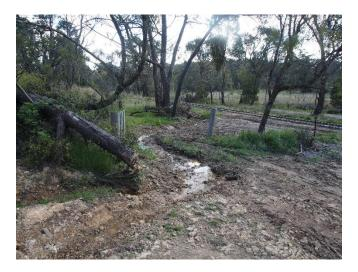
Water flow off Black Bullock Road has been diverted into rail corridor and under the track to stop the new rail crossing from damage
