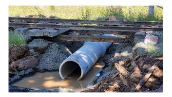
Rebuilding drainage on the track. After 100 years this culvert had completely deteriorated. Photo shows engineering of times past with rail supporting the track over the culvert.
