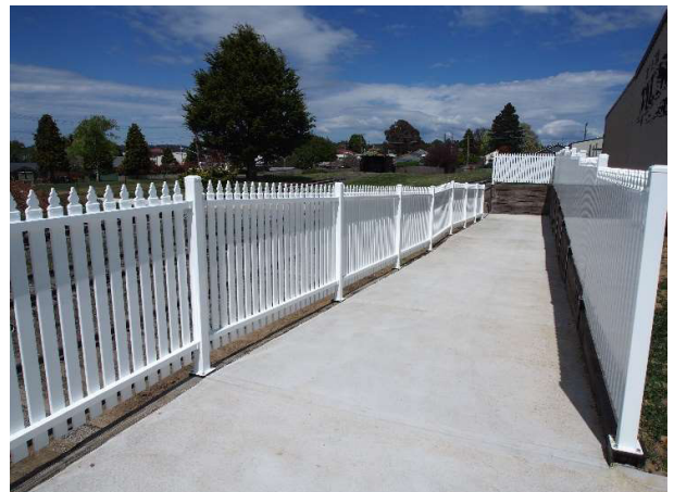
New pathway showing the safety fence.
