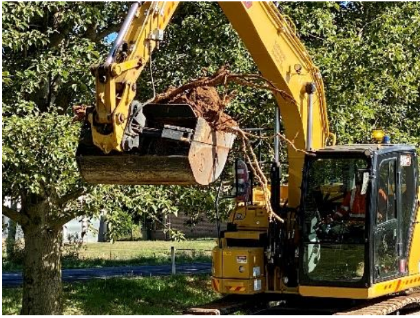
Preparing the pathway for the railway
