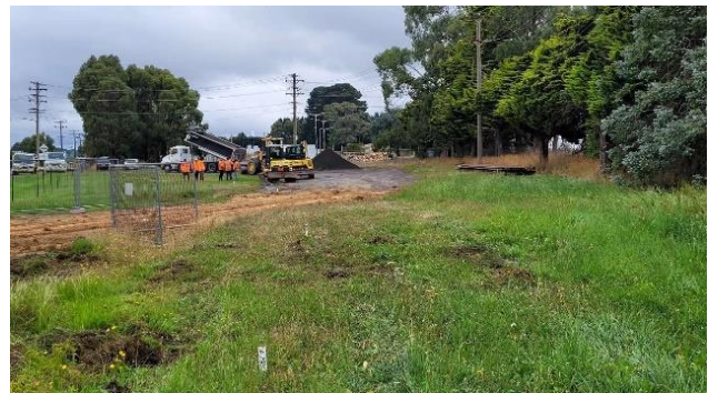
Survey pegs ready for the new piece of railway line in Lowes Mount Road with preparatory work in the background.
