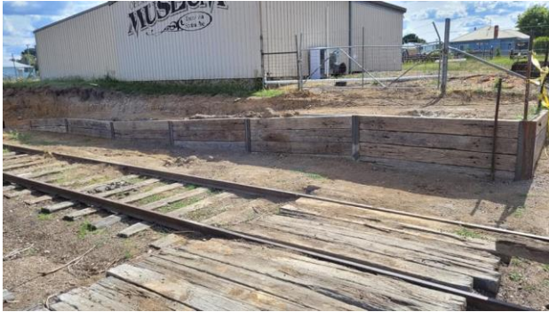
Reinforced wall under construction
