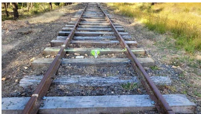
Survey peg in position for the North end righthand turnout
