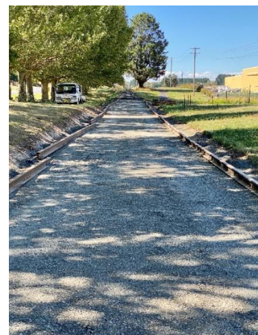
Preparing to lay line.
