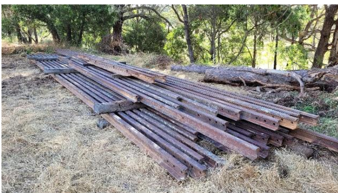
Rail stored in readiness for the building of the turnaround loop.
