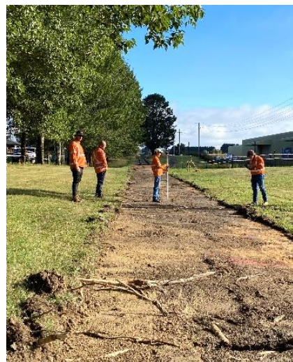
Surveying the track-
