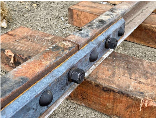
Brand new fish plates as well as new nuts and bolts - obviously yet to be pinned
