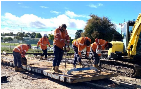
CAM workers preparing sleepers for laying on the track
