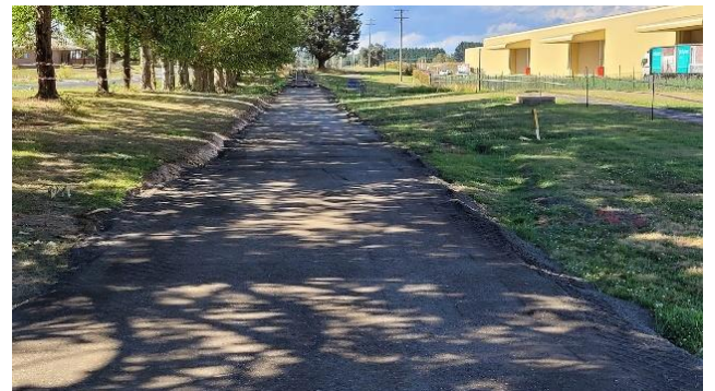
Earthworks outside the Borg factory looking South towards Oberon.
