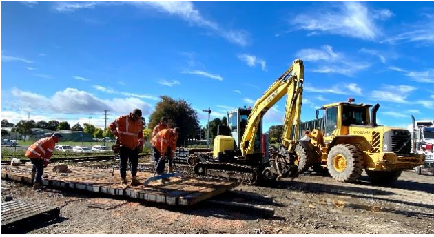
CAM workers preparing sleepers for installation of the lost 1/2 kilometre.
