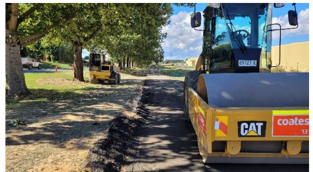
Compacting the base ready to receive the line.
