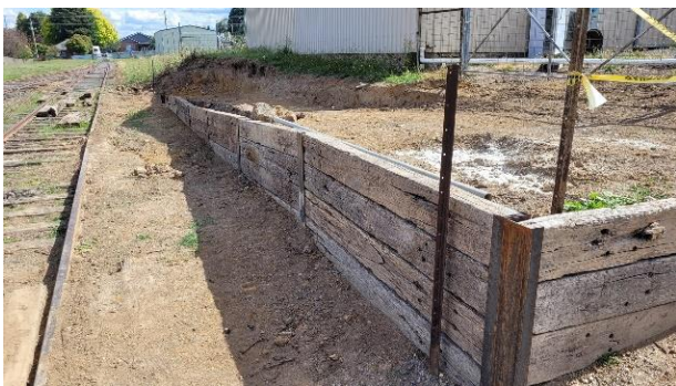
Another angle showing the retaining wall.
