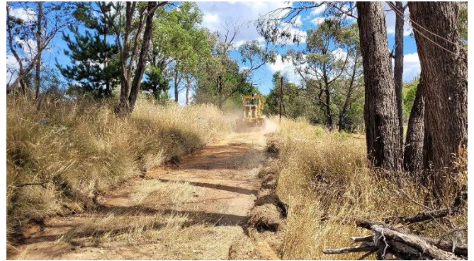
Grading of the access track south of Black Bullock road
