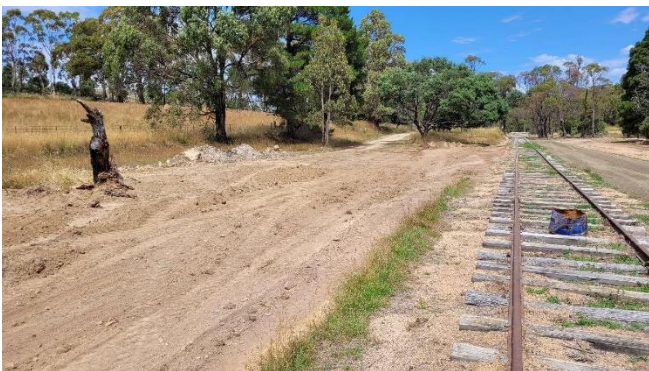
Earthworks at the levelled site for the new Hazelgrove station.
