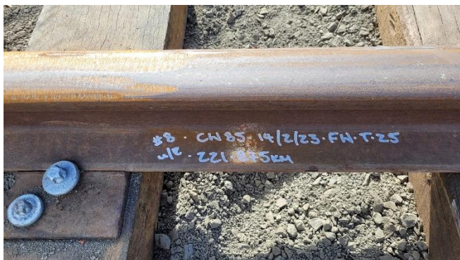
Close up photo of workmanship on new track.
