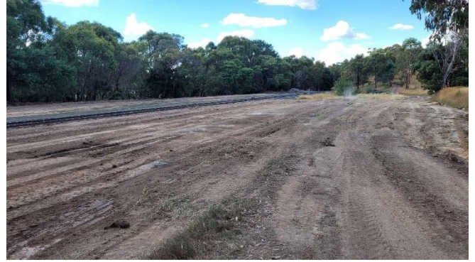
Eastern side of the track site preparation
