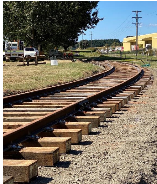
Part of the “missing link” now back in place.
