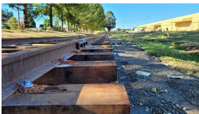
A ground view of the new track.
