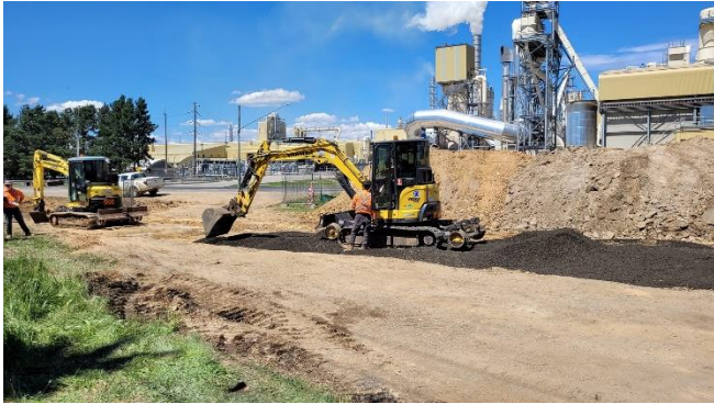
Base laid down on prepared path.
