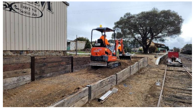
Preparation in progress prior to laying the concrete path
