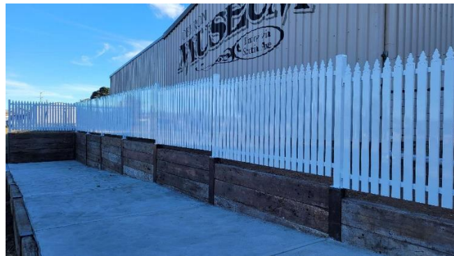
A closer aspect of work done to date.
