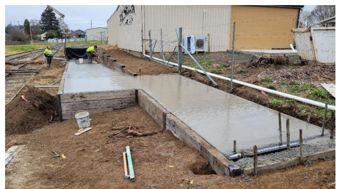
The team from J & H concreting finishing the concrete
