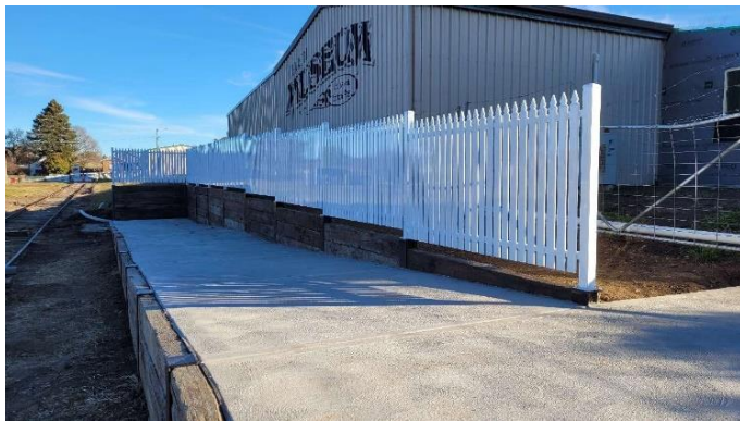
The finished path with some fencing in place.
