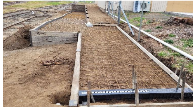
Reinforcement in place
