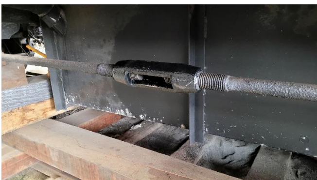
HLF854 truss rod and turnbuckle fitted and adjusted.
