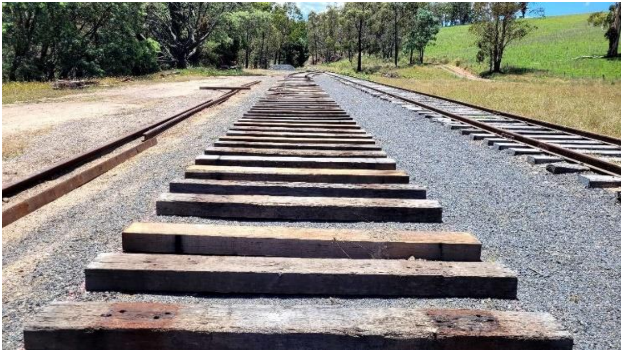
Sleepers laid in place as surveyed, looking North.
