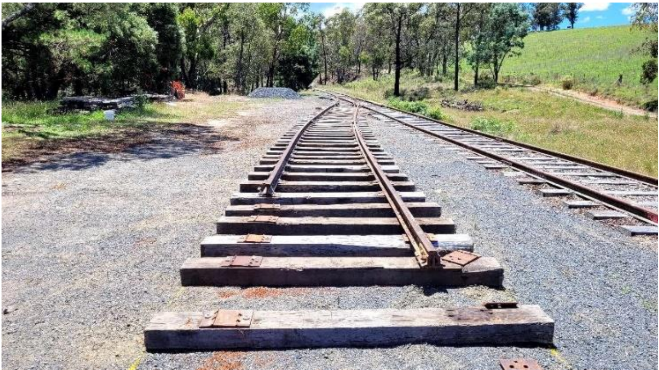
Looking back to the north showing commencement of the loop line.
