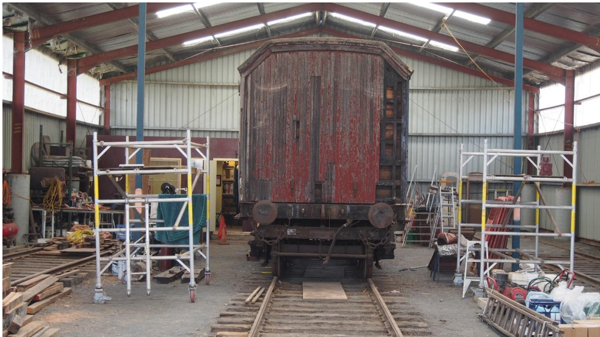
February 1 st HS36 was moved to the middle road of the rolling Stock shed
