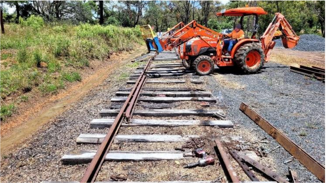
Line being removed by OTHR Volunteers to accommodate the Southern Turnout
