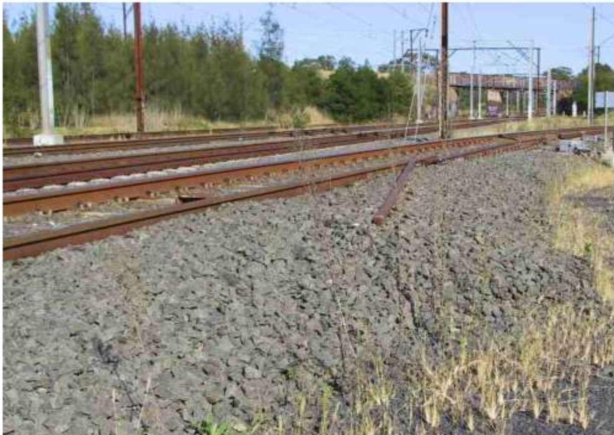
Figure 3 – Example of catchpoint with poor landing zone
