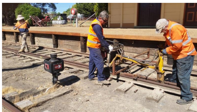
Volunteers replacing the line in front of the station at the last working bee.
