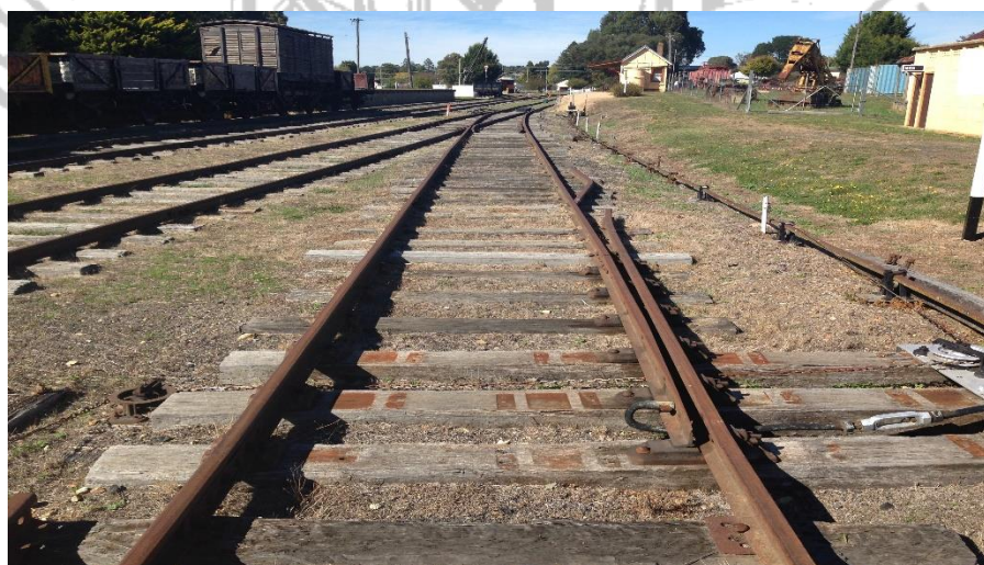
Catchpoints controlled by Lever 2 at the "B" frame
