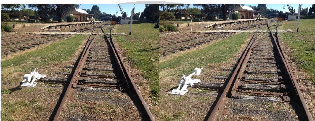
Points changed by a 'Throw over' lever
