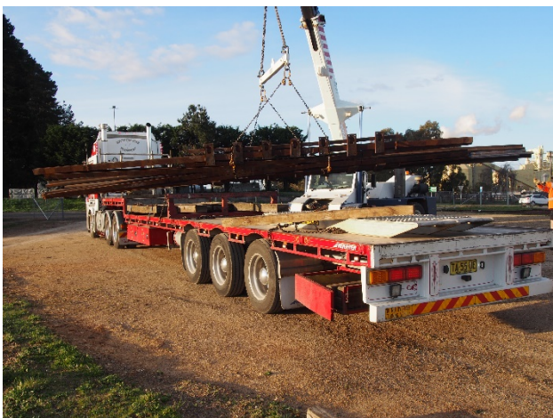
Unloading the turnout materials received from Gilgandra, NSW
