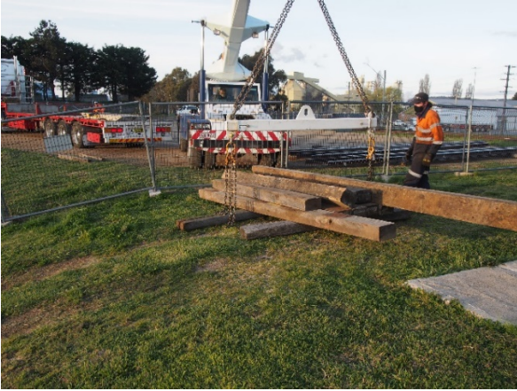
More turnout materials unloaded to the Oberon Storage Yard.
