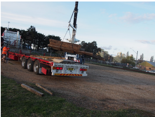
New turnout arrives at Oberon Storage Yard
