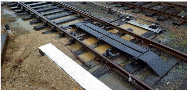
Problem: erosion of station and pooling of water.
