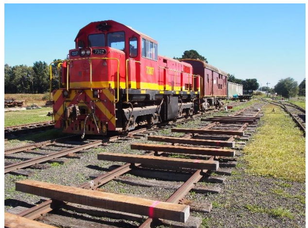
Photo taken on January 16 th during the shunt The new sleepers on road 2 have replaced old sleepers at the end of their useful life in road 3
