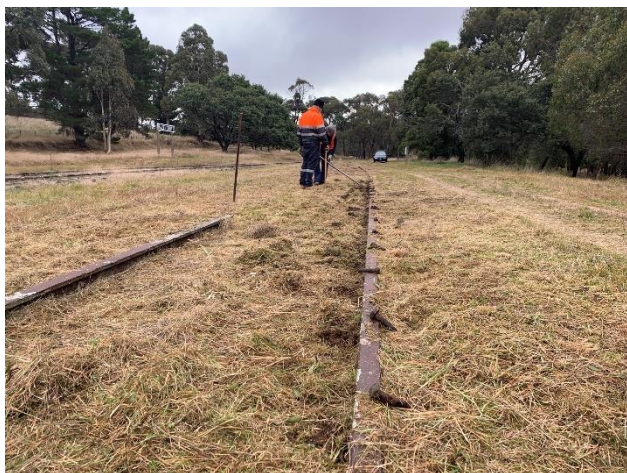
De-pinning at Hazelgrove. Many dog spikes could be removed by hand
