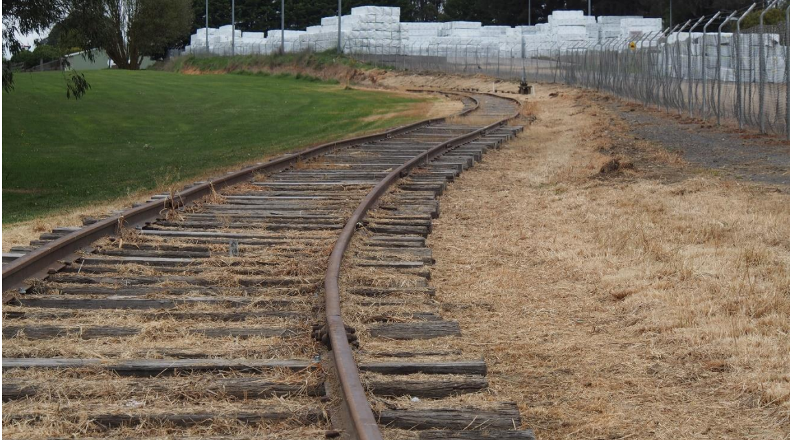
Completed - Spraying and whipper snipping on the track near Highland Pine Note that the fence has been moved back to improve train clearance
