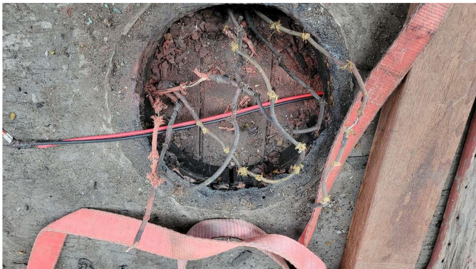
Old lighting wiring above guard compartment below roof vent.
