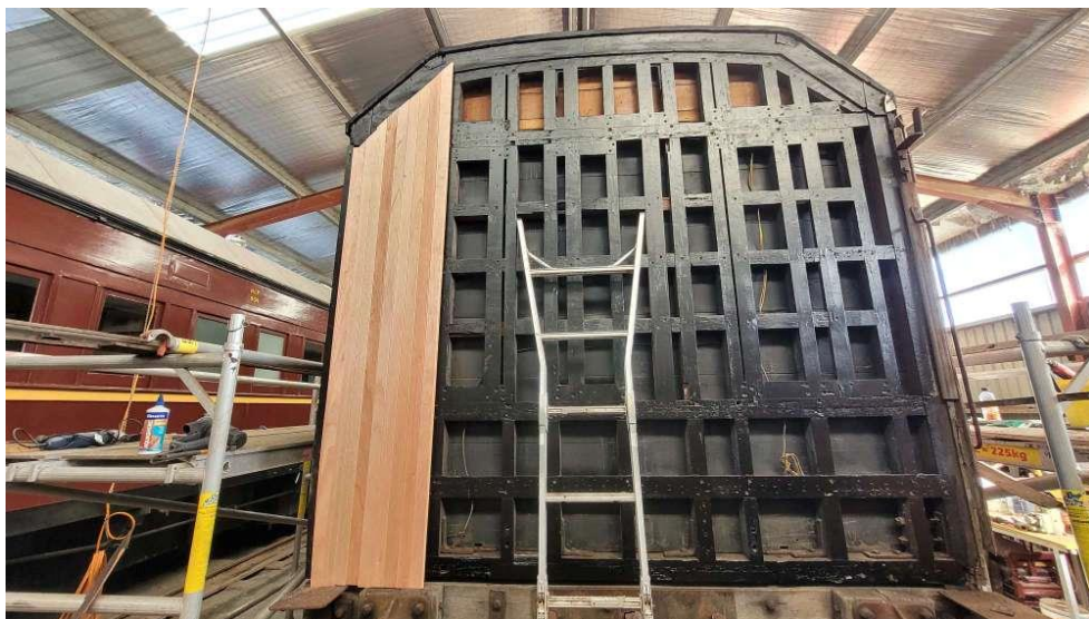
Matchboard application guard end.
