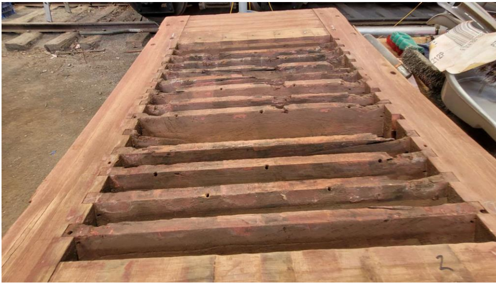
Dogbox door work. Note dog chew marks on louvers.
