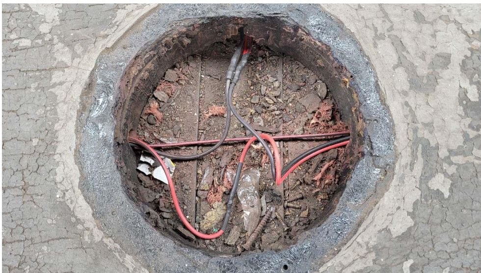
Old lighting wiring above guard compartment below roof vent.
