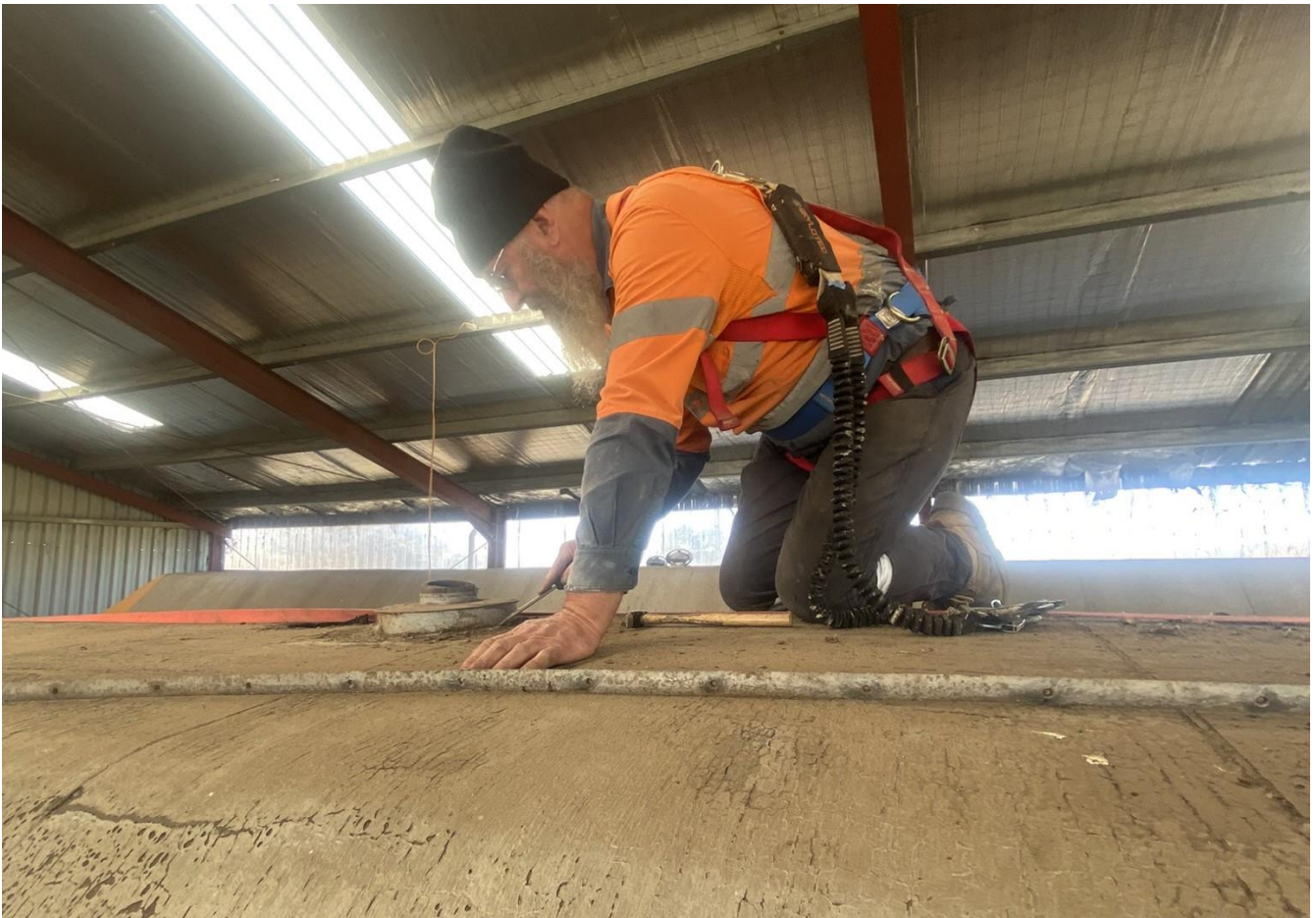
Michael Clark – HS36 Project Manager removing damaged roof vents for repair.
