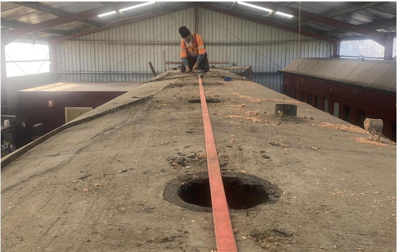
Michael Clark removing roof vents for repair on HS36
