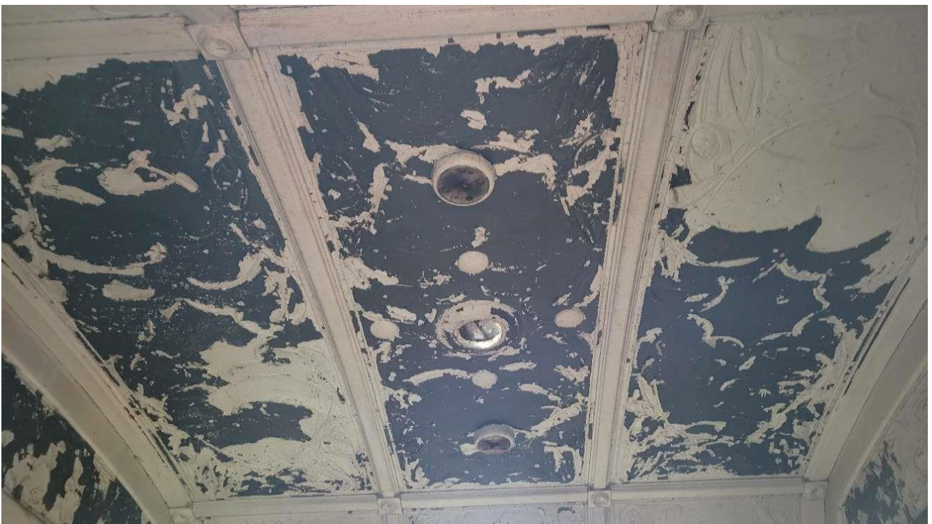
1 st class ceiling before laser cleaning.
