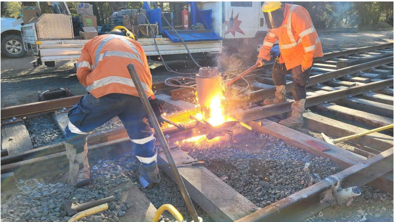
Thermite welding. Hot stuff!
