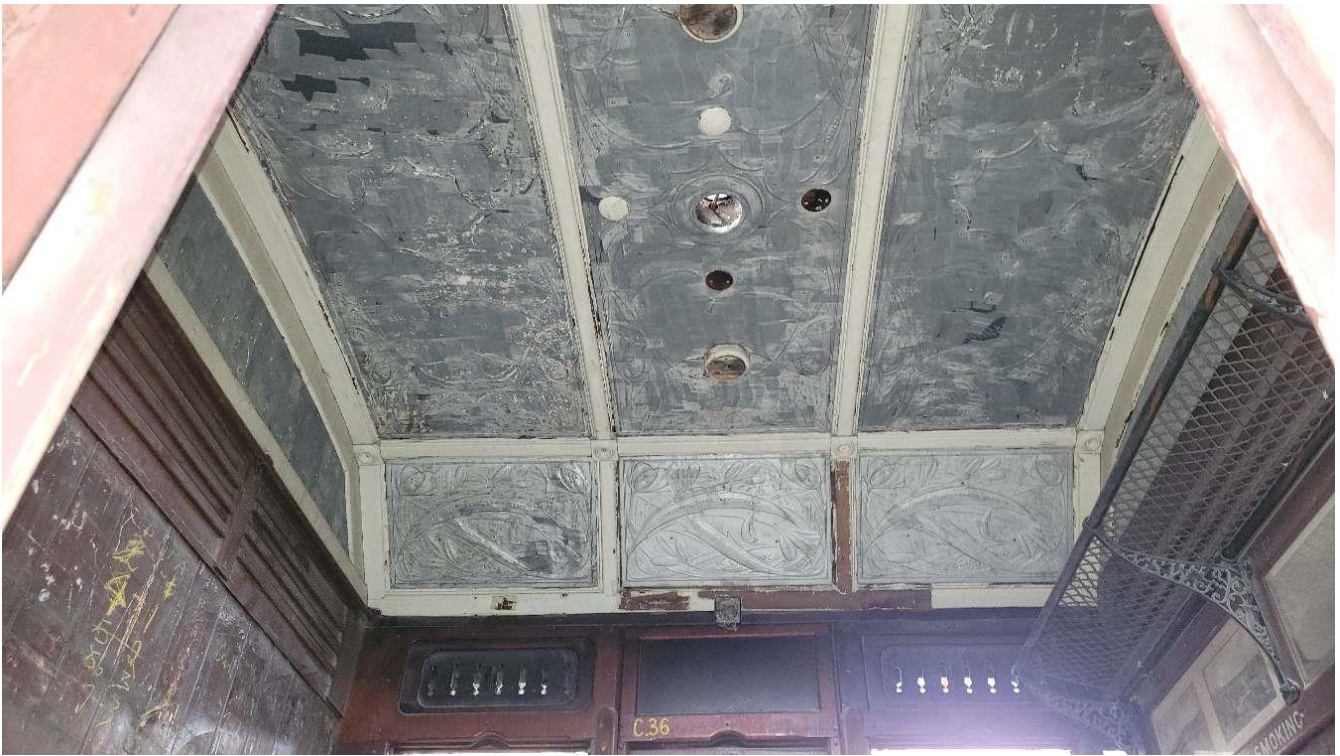
Ceiling after laser cleaning
