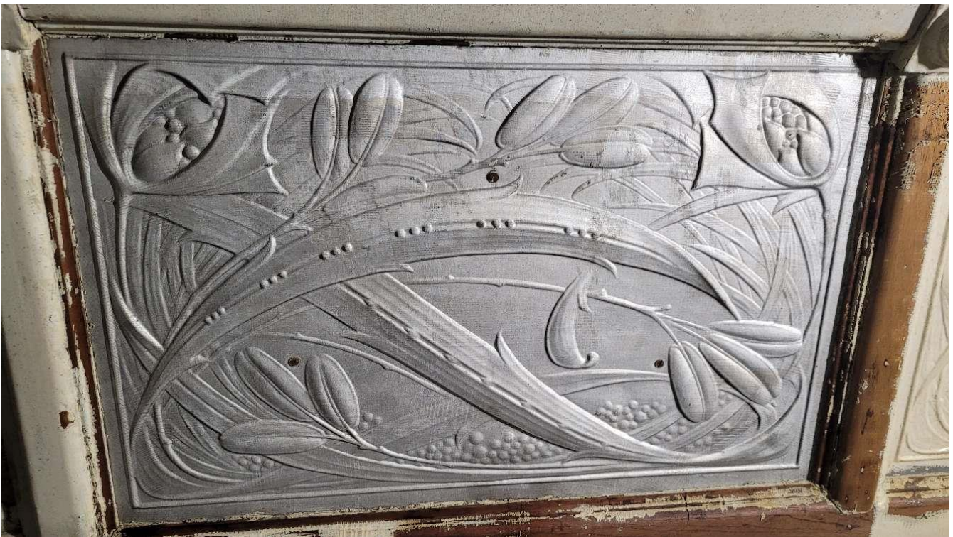
Close up of one of the laser cleaned panels in first class almost ready for paint.
