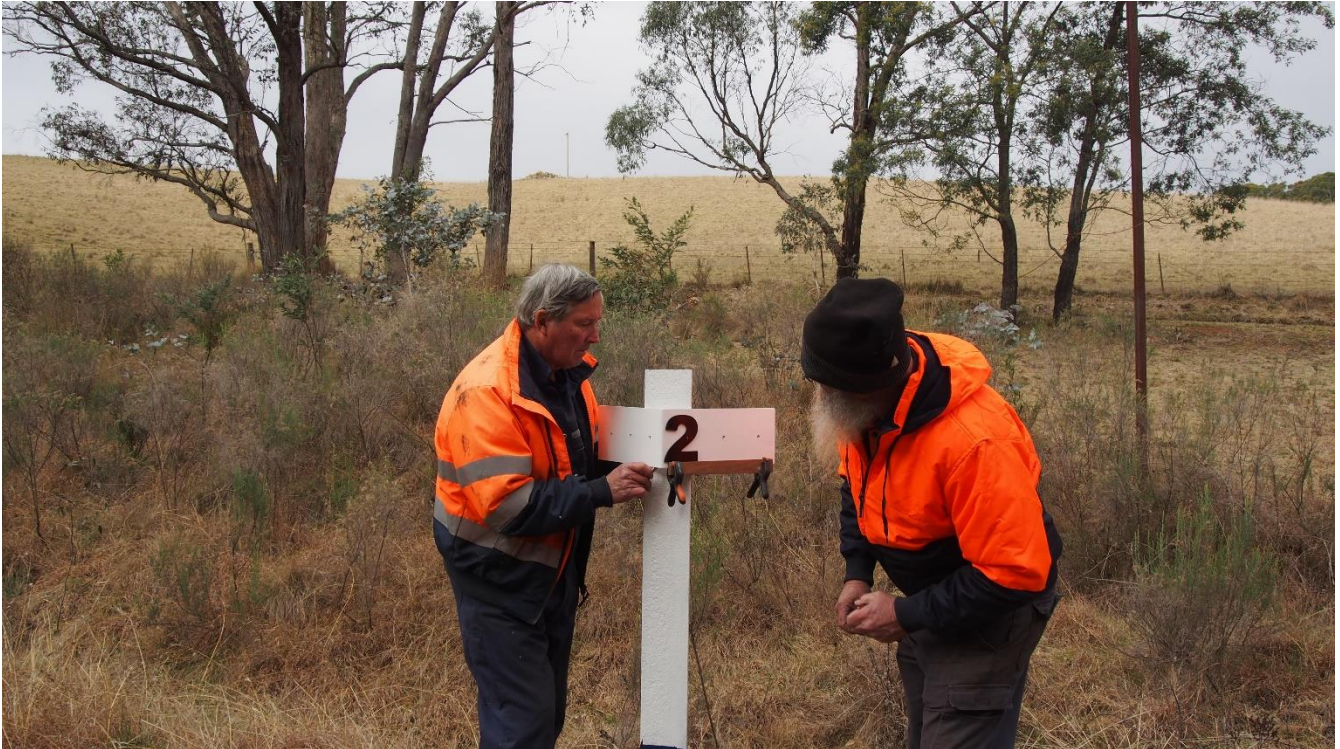
Finishing the 217 Kilometre Post just south of the stop block at Hazelgrove
