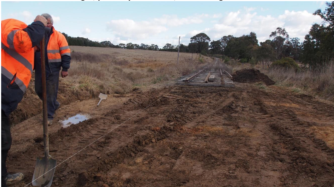
End of Day Track Work 23 rd August At 218.600 12 sleepers removed 3 lengths of rail removed
