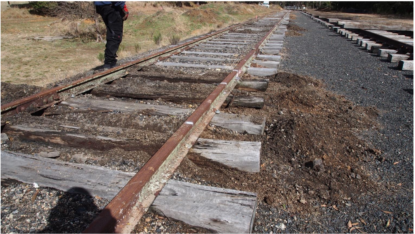
Some of the older sleepers at Hazelgrove, dog spikes out and ready for removal
