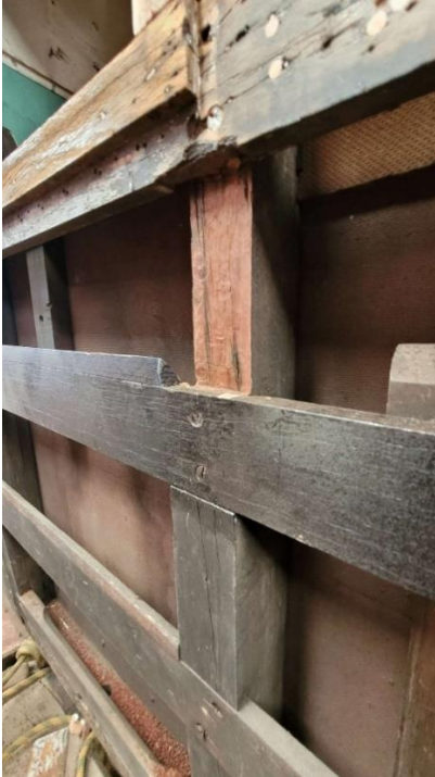
Rot cut out down to good timber
