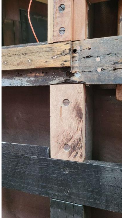
New timber spliced in
