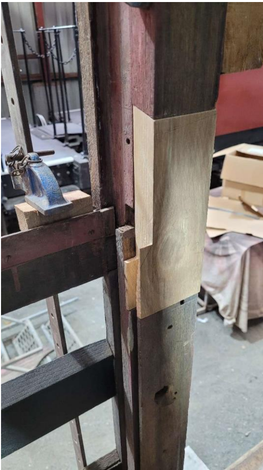
Frame repaired (awaiting fastening)
