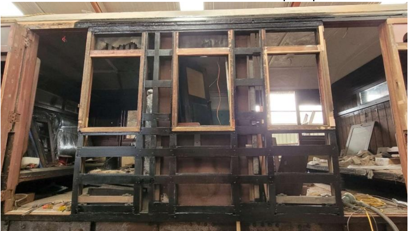
C36 to D36 frame complete and painted ready for cladding.
