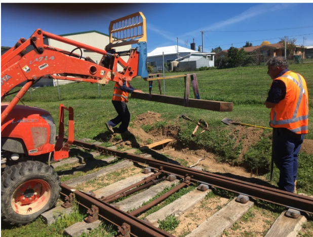
Placing the timber for E-frame - March
