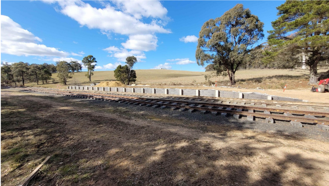
Hazelgrove West Platform Wall Taking Shape
