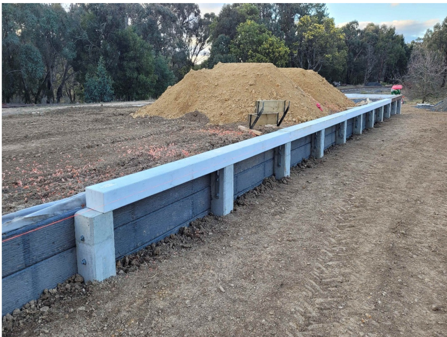
First coping timbers placed
