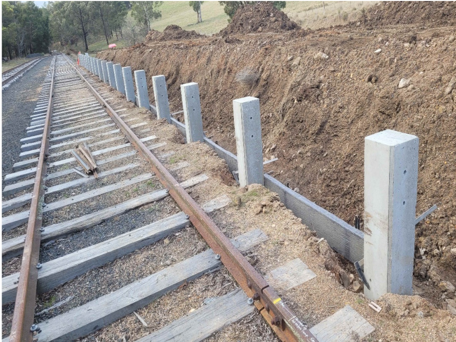
First course west wall retaining rails in place
