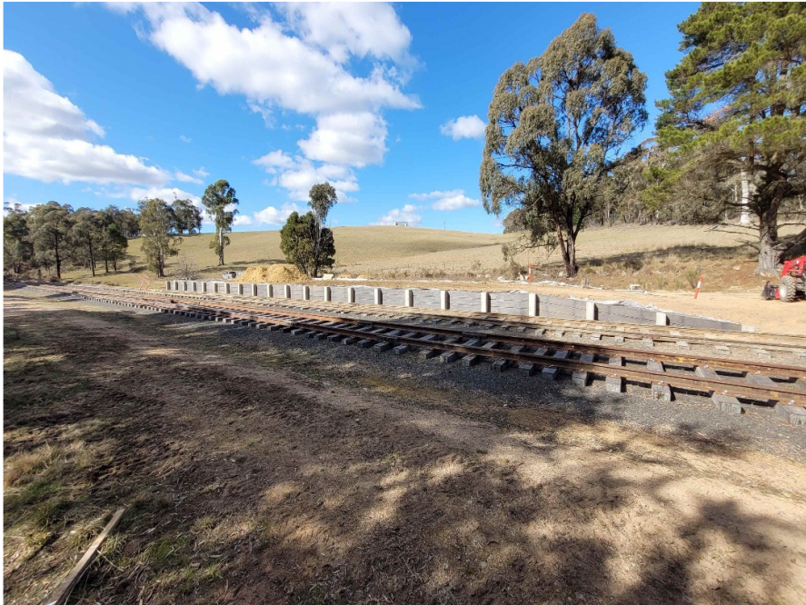
West wall, all retaining rails in place
