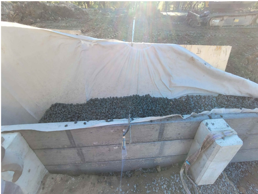
Geo cloth and aggregate being placed
