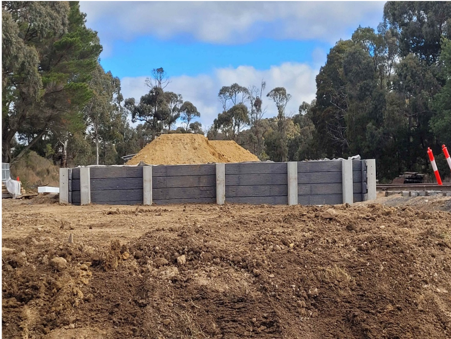
North wall rails placed
