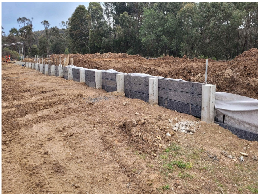
East wall retaining rails being placed
