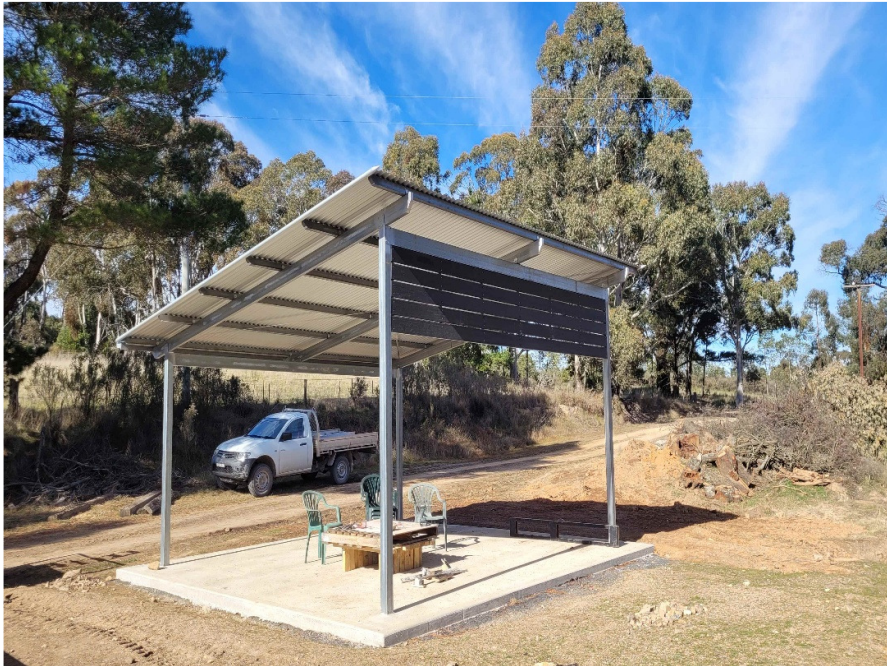
Picnic shelter structure completed
