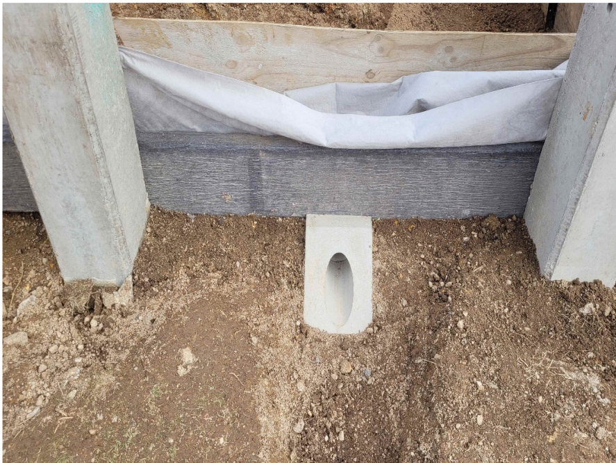
North wall ag drain exit
