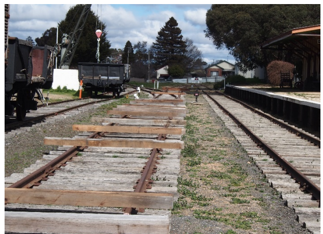
Sleepers in place ready for work on road 3 in front of the station
