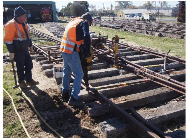
Hammering in the dog spikes
