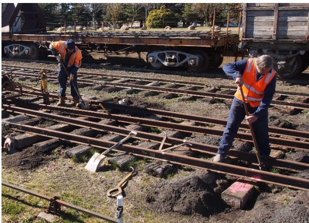
Graham and Mark on the end of a shovel replacing timbers at Micro-working bee in July
