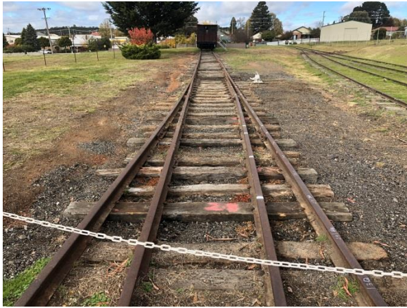
PWD's siding showing new timbers working bee 2 nd May
