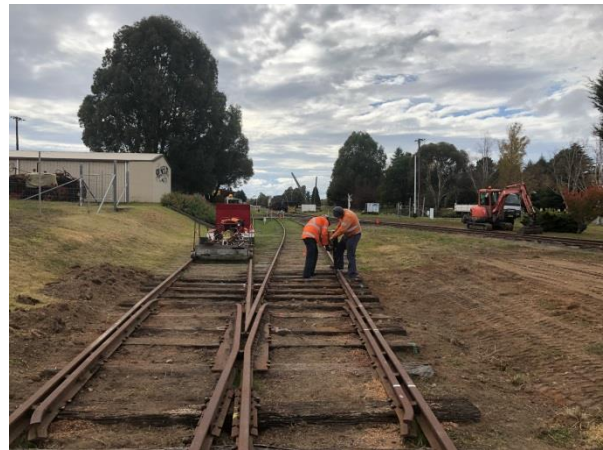
Last dog spike driven in on that part of the job. Volunteers working bee 2 nd May
