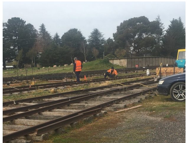
A couple of fettlers – checking road 4 In gauge? Is it level?
