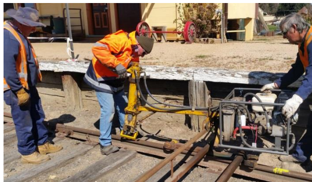
Not quite pulling teeth! Our volunteers using the dog spike puller. Working Bee September/October.
