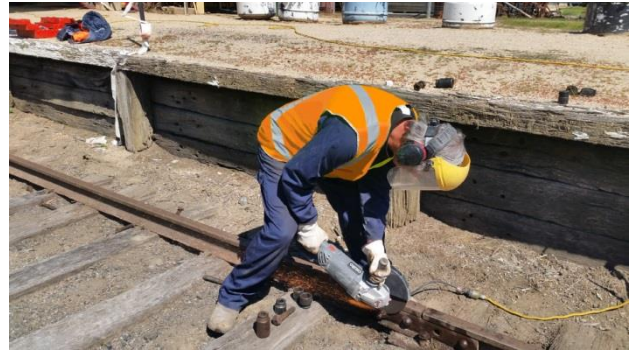
The hard grind! One of our volunteers readying the rail for replacement. Working Bee September/October
