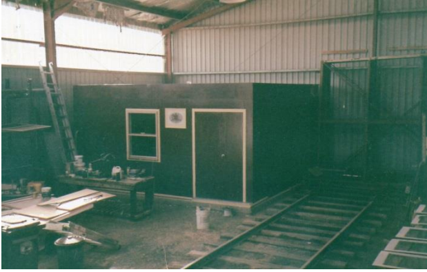
OTHR's new storage room located within the rolling stock shed. This was a project of the working bees of the past three or four months.
