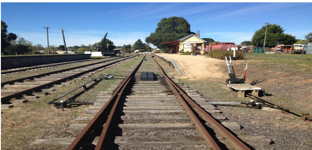
Frame points controlled by the lever 1 frame 'B' on the right
