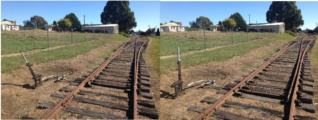
Points changed by a 'Ball' Lever
